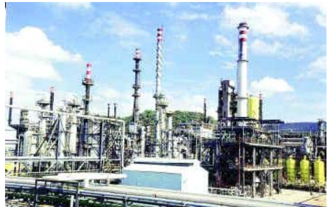
HPCL's refinery in Visakhapatnam, India
